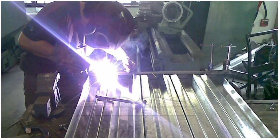
Figure 5.4 Welding of the C channel to the Peva 45
