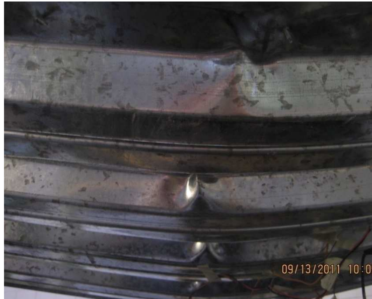
Figure 5.17 Local buckling in the profiled steel sheeting
