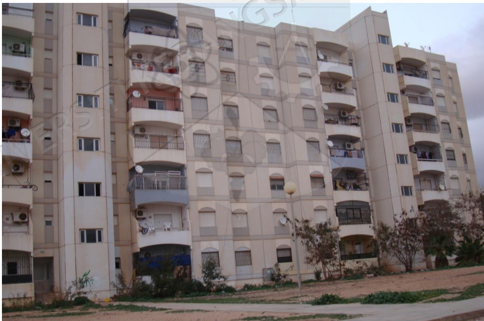
Photo 3.4 A six story building in Al-Keesh area
