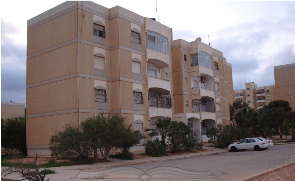
Photo 3.3 A four story building in Al-Keesh area
