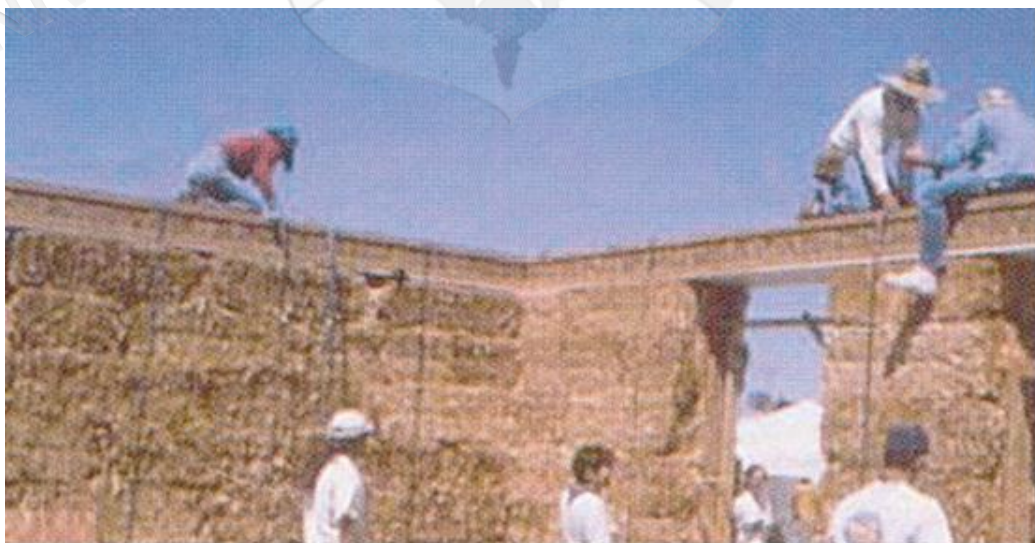
Photo 3.5 Building hay houses
